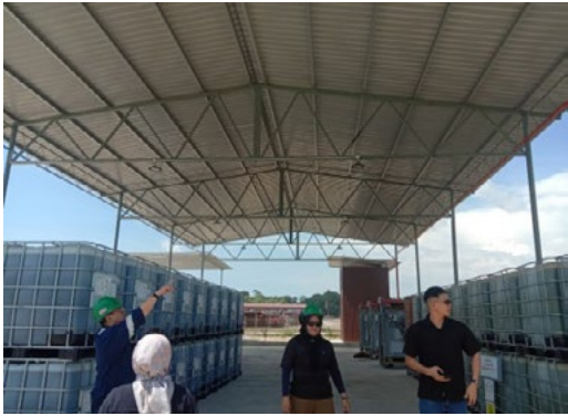
A Partnership Built on Safety: Altus & SSTCM in Labuan 18
